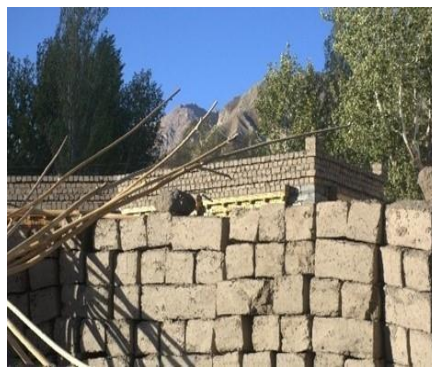
Figure 6 (a): Traditional Façade (b) Sun-dried Earth Block (c) Traditional ceiling [23]
