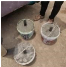
Figure 13: Bucket Foundation
