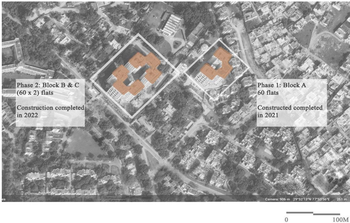
Figure 2: Apartment complex consisting of the case study building
