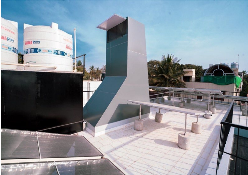
Figure 2: Photo showing the constructed Solar Chimney
