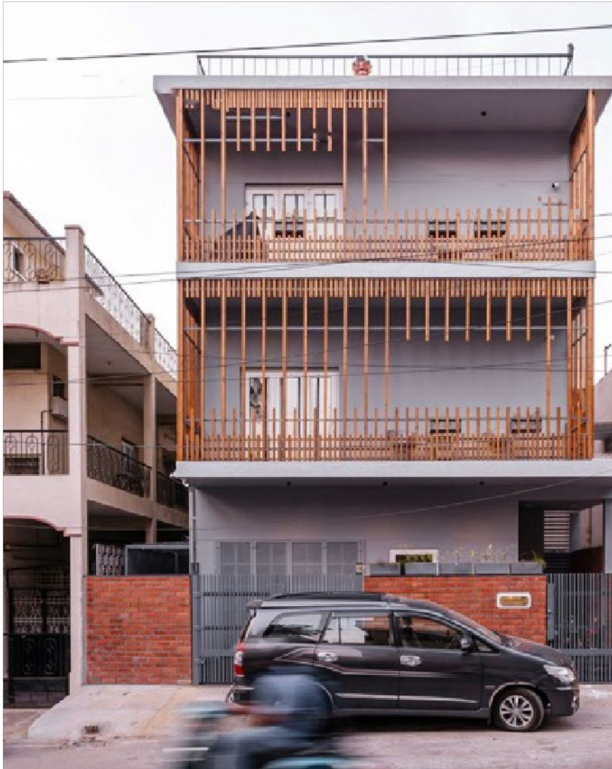
Figure 5: Image of the house after renovation and retrofit, 2023
