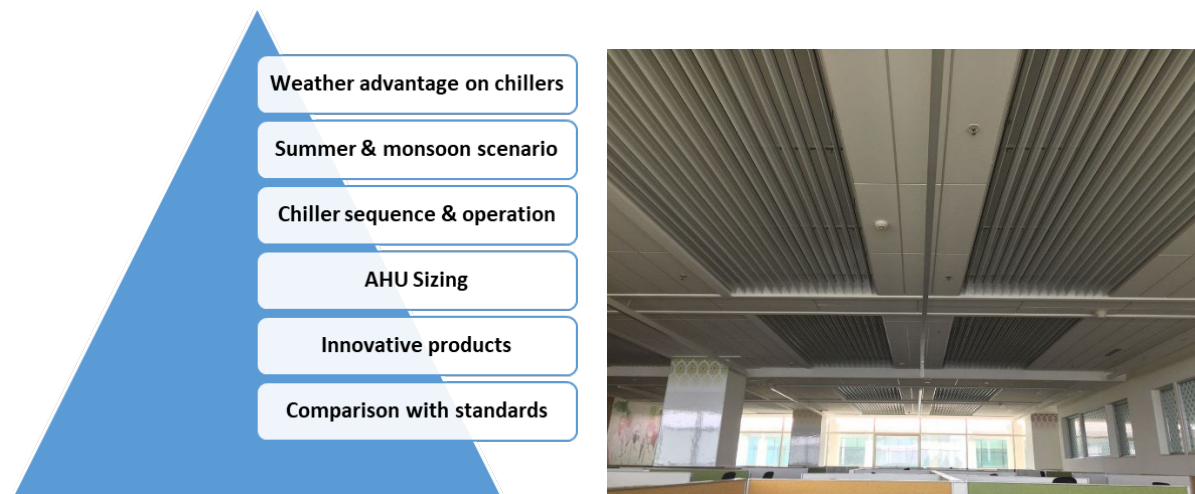
Fig 8: HVAC design innovation
