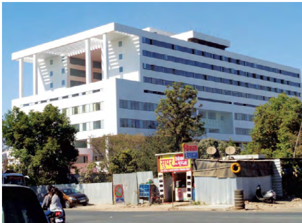
Figure 1: Hospital Building, Pune
