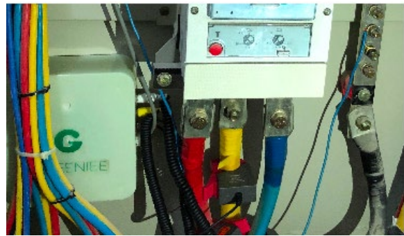
Figure 4: Picture of actual installation of Greeniee
