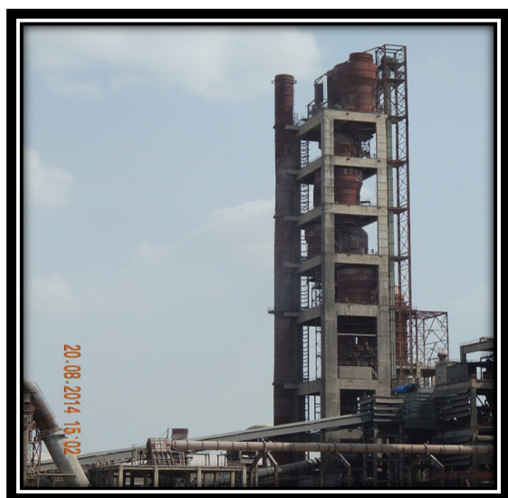
Figure 4: 6 STAGE PREHEATER
