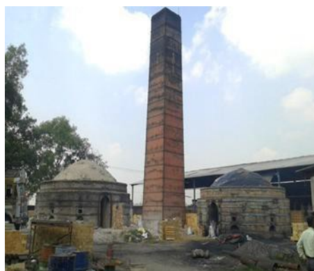
Figure 2: Downdraft kiln
