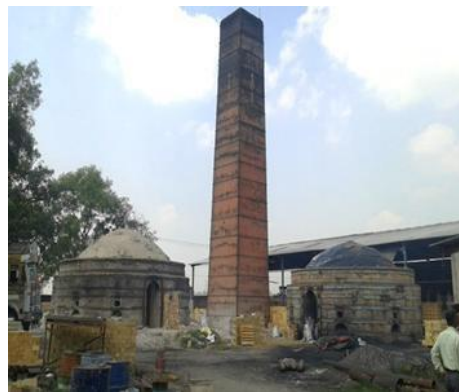
Figure 2: Downdraft kiln
